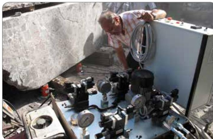
*Hydraulic pump with 4 independent outlets for synchronous lifting of the load, independently from the different load weighing on each cylinder.*
