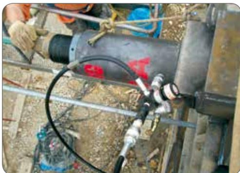
*Hollow, single-acting cylinder with safety ring CRM 60/260 GS for bridge launching operations.*
