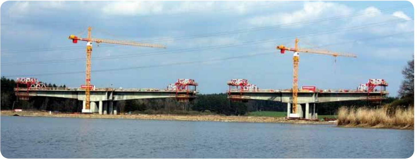
The gradient of the bridge was achieved with cantilevered cranes, launched using a hydraulic F.P.T. system complete with double-acting cylinders with locking ring, hollow cylinders and hydraulic pump to launch 4 complete carts, 2 for each pier.
