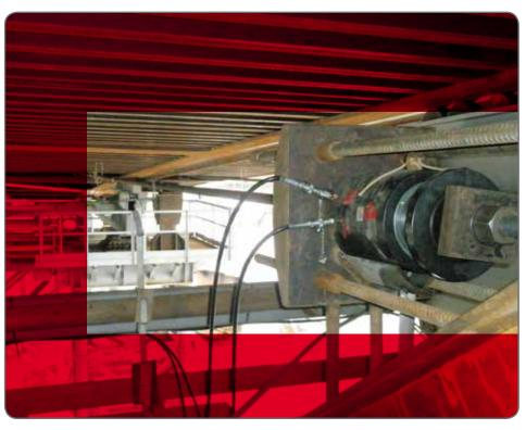
Road bridge movement and levelling on pier using 8 hollow, 60-ton cylinders.
