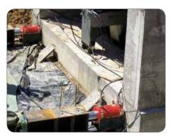
CRIC 250/250 cylinders for shifting a prefabricated concrete structure.
