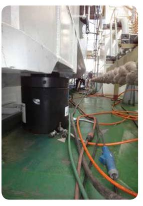
4 high-tonnage double-acting cylinders, with 600 ton-capacity 250 mm flow mechanical locking ring, controlled by 2 F.P.T. hydraulic pumps.
