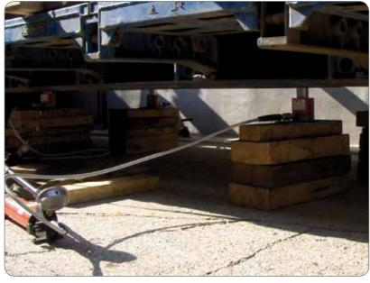
Compact cylinders F.P.T. model - CRM50/50C controlled by two-speed PDSA21 hand pump to level a structure
