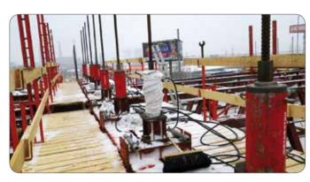
Lifting sections of concrete structure bridges using 60 ton-capacity hollow cylinders and traction bars.
