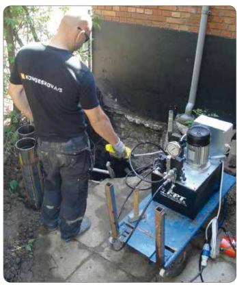
Hydraulic pump with solenoid valve and 20 I tank.
