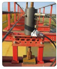
CRI 100/150 FO and CRI 60/250 FO GS cylinders used for lifting structures in the infrastructure sector.
