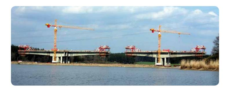
The gradient of the bridge was achieved with cantilevered cranes, launched using a hydraulic F.P.T. system complete with double-acting cylinders with locking ring, hollow cylinders and hydraulic pump to launch 4 complete carts, 2 for each pier.
